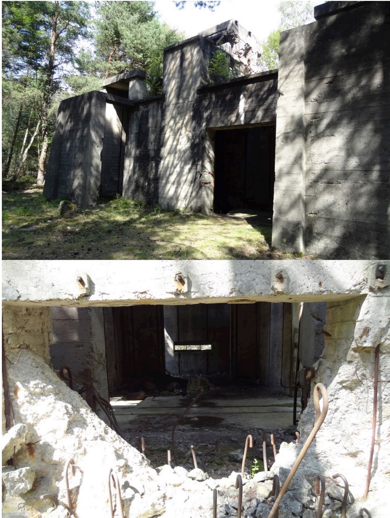
Figure E.40: Historisch-Technisches Museum Versuchsstelle Kummersdorf: Rocket engine test building large enough to accommodate test firings of A-4 engines (upside down with the exhaust vented through the roof).
