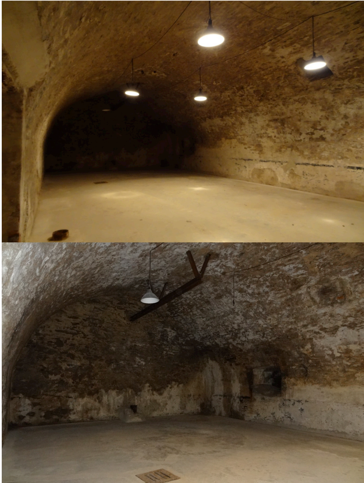
Figure D.397: The former Atomkeller in Stadtilm. In the lower photo, note the circular pit in the floor, now filled in with concrete, which once held the heavy water with uranium cubes suspended in it from the overhead beam.
