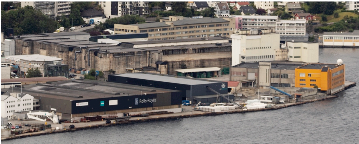
Figure 7.129: The U-boat bunker Bruno in Bergen, Norway could hold and service up to nine submarines at a time, with six meters of overhead concrete reinforcement to protect them from Allied aerial bombing.
