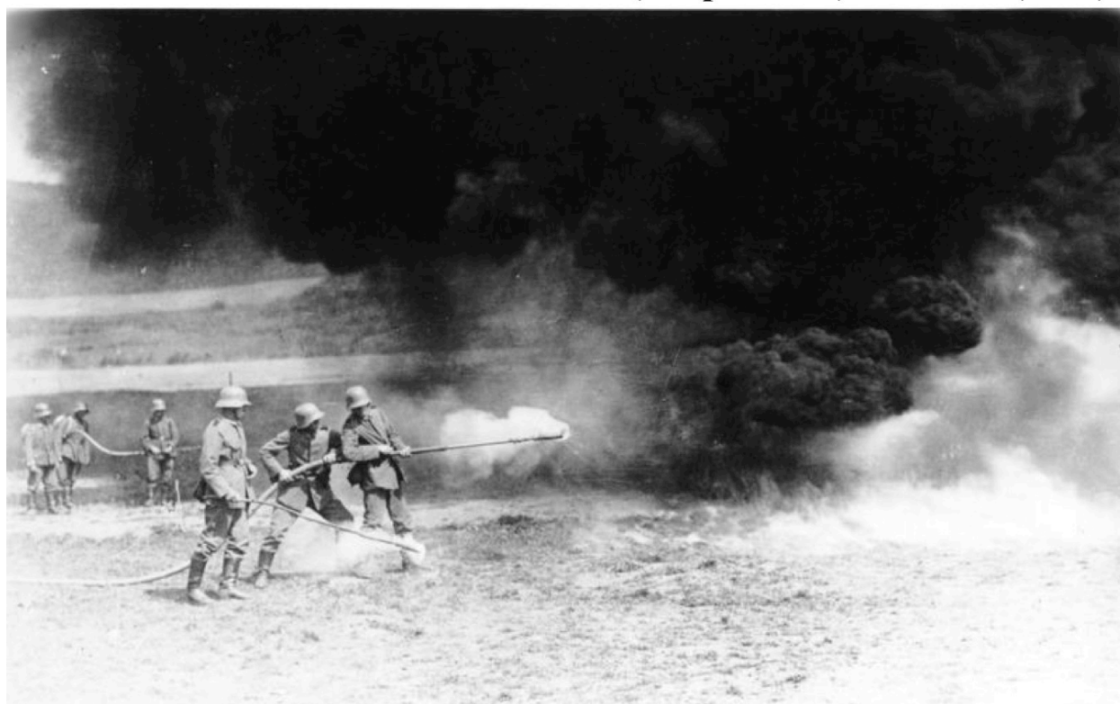
Figure 7.104: Richard Fiedler invented the modern flamethrower in 1901 and developed improved versions until 1918. Bernhard Reddemann and Gábor Szakáts began developing improved flamethrowers in 1904 and 1915, respectively. The Grossflammenwerfer (Grof, 1912) had a fixed (nonportable) fuel tank, required a crew of three operators, and had a range of 35 meters.
