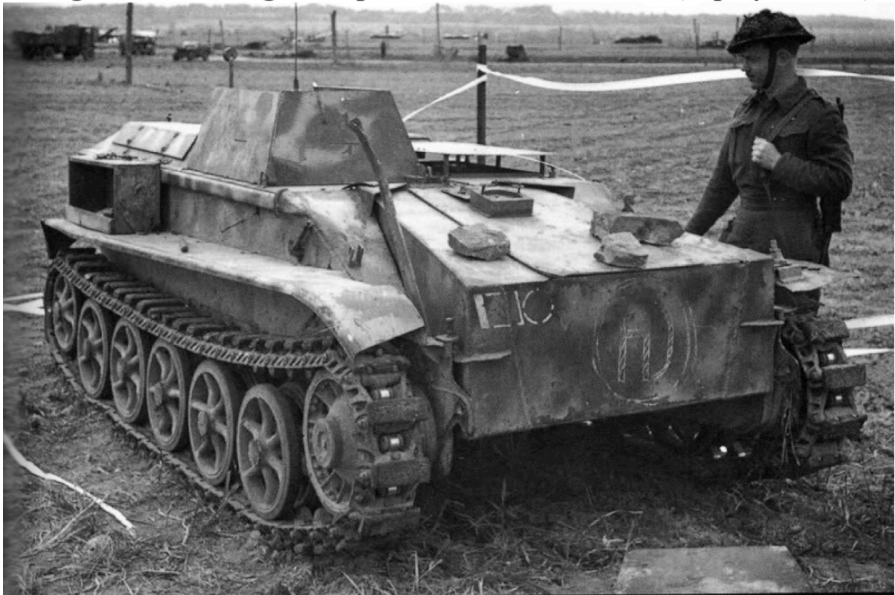
Figure 6.196: Larger teleoperated battlefield robots that were used in combat by Germany included the Mittlerer Ladungsträger Springer and the Schwerer Ladungsträger Borgward B IV.
