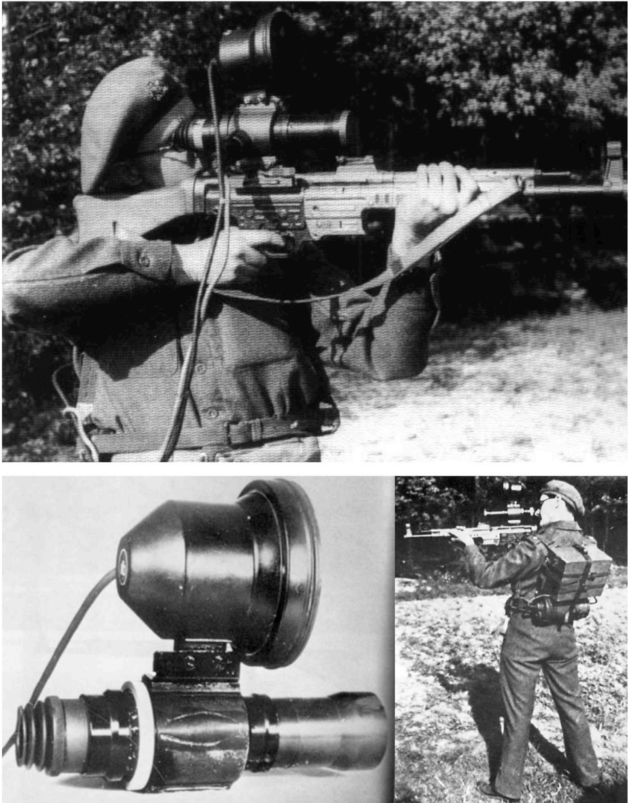
Figure 6.144: The Zielgerät 1229 Vampir (Vampire) infrared night-vision system for snipers, first operational in 1944 [BIOS Misc 66].
