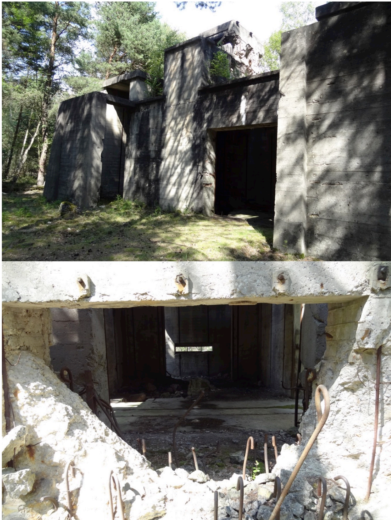
Figure E.29: Historisch-Technisches Museum Versuchsstelle Kammersdorf: Rocket engine test building large enough to accommodate test firings of A-4 engines (upside down with the exhaust vented through the roof).
