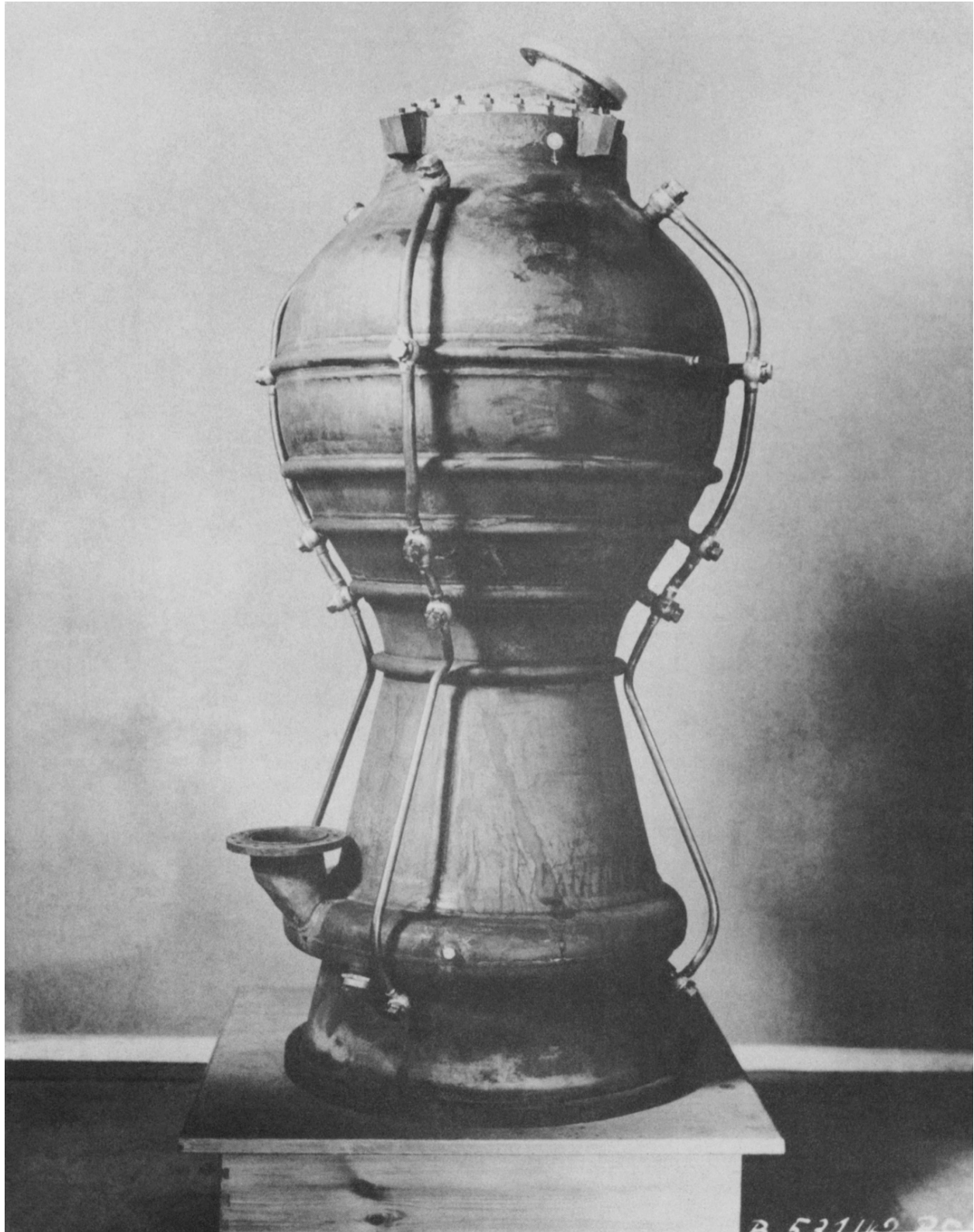
GERMAN A-4 ROCKET COMBUSTION CHAMBER (PRODUCTION)
