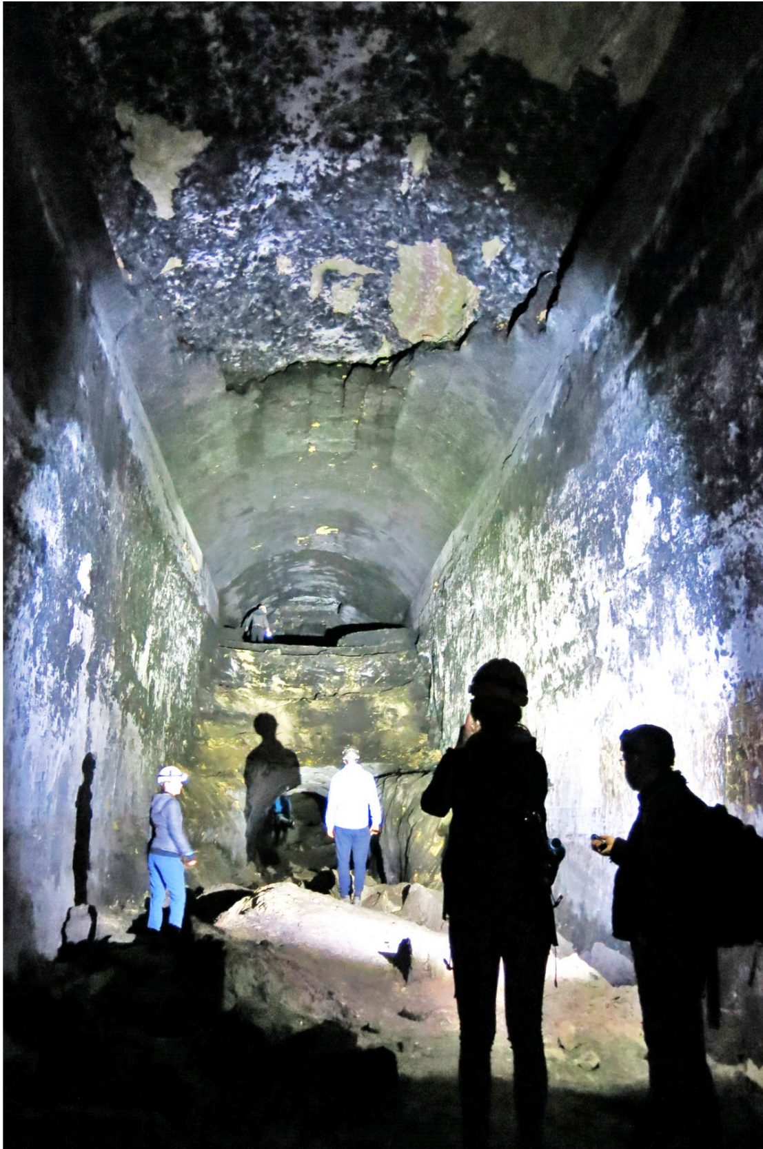
Figure E.15: Remains of the huge underground factory for Me 262 jet fighters at Kahla [photo courtesy of Frank Döbert].
