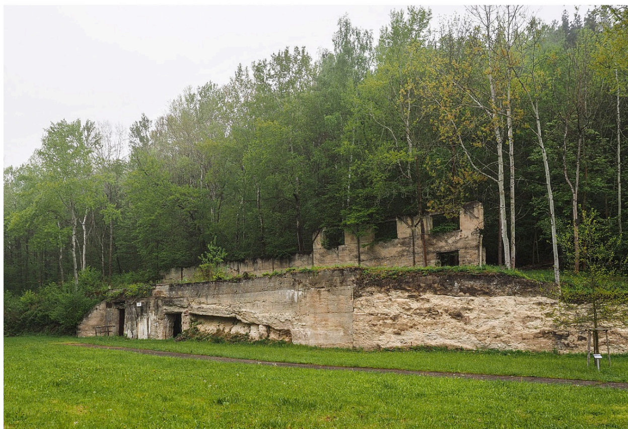
Figure E.13: Remains of the huge underground factory for Me 262 jet fighters at Kahla.
