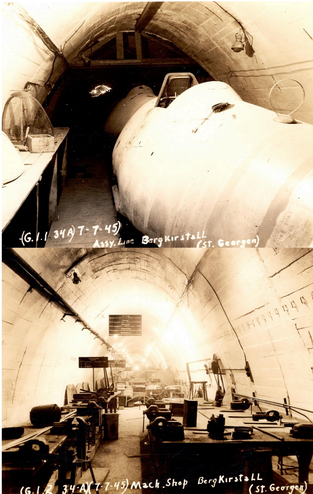
Figure D.963: More photos taken by U.S. soldiers at the Bergkristall tunnel complex at St. Georgen an der Gusen in May 1945 [AFHRA 00043922 SQ-BOMB-34-HI 1-31 July 1945].
