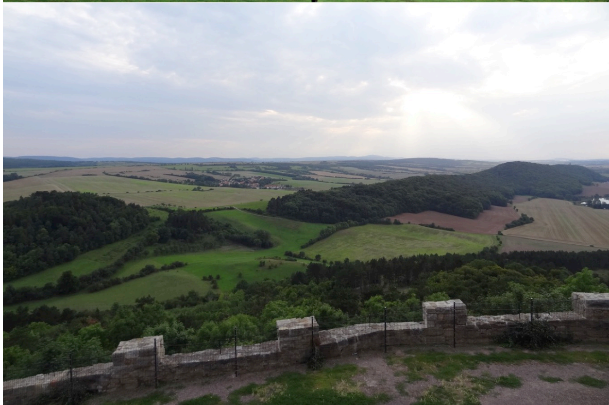
Figure D.736: Wachsenburg castle now, and the view from the castle of the village of Röhrensee and beyond.
