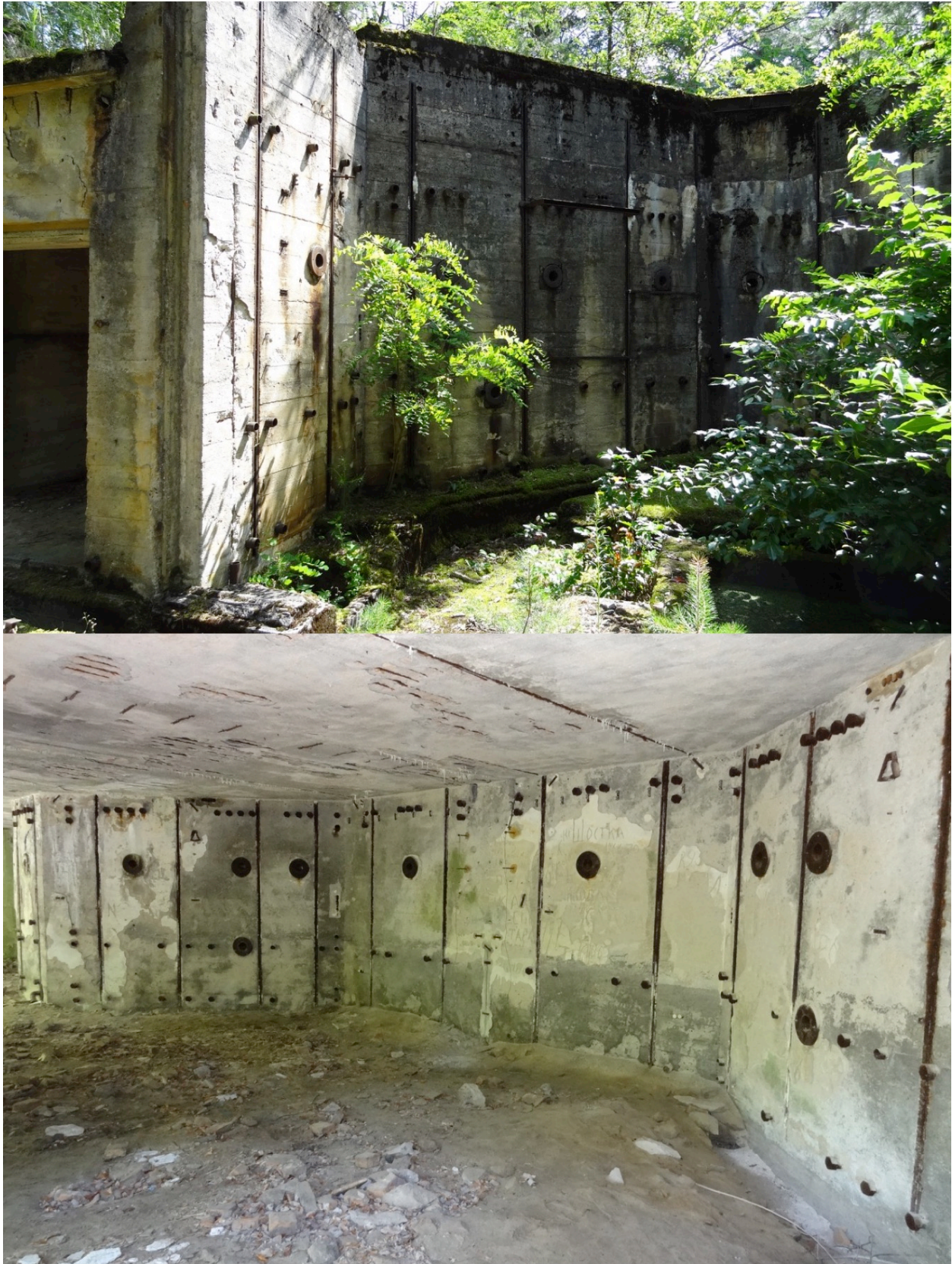
Figure D.562: Historisch-Technisches Museum Versuchsstelle Kummersdorf: Apparent testing area for implosion designs; note numerous ports for mounting diagnostic equipment.
