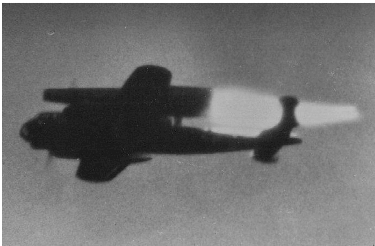
Figure 9.100: Eugen Sänger's ramjet being tested on a Dornier Do 217 aircraft (1942).
