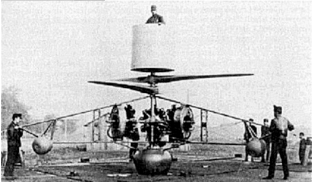
Figure 9.125: István Petrőczy, Theodore von Kármán, and Vilém Žurovec created proto-helicopters such as the electric-powered PKZ-1 (1918) and gasoline-powered PKZ-2 (1918).
