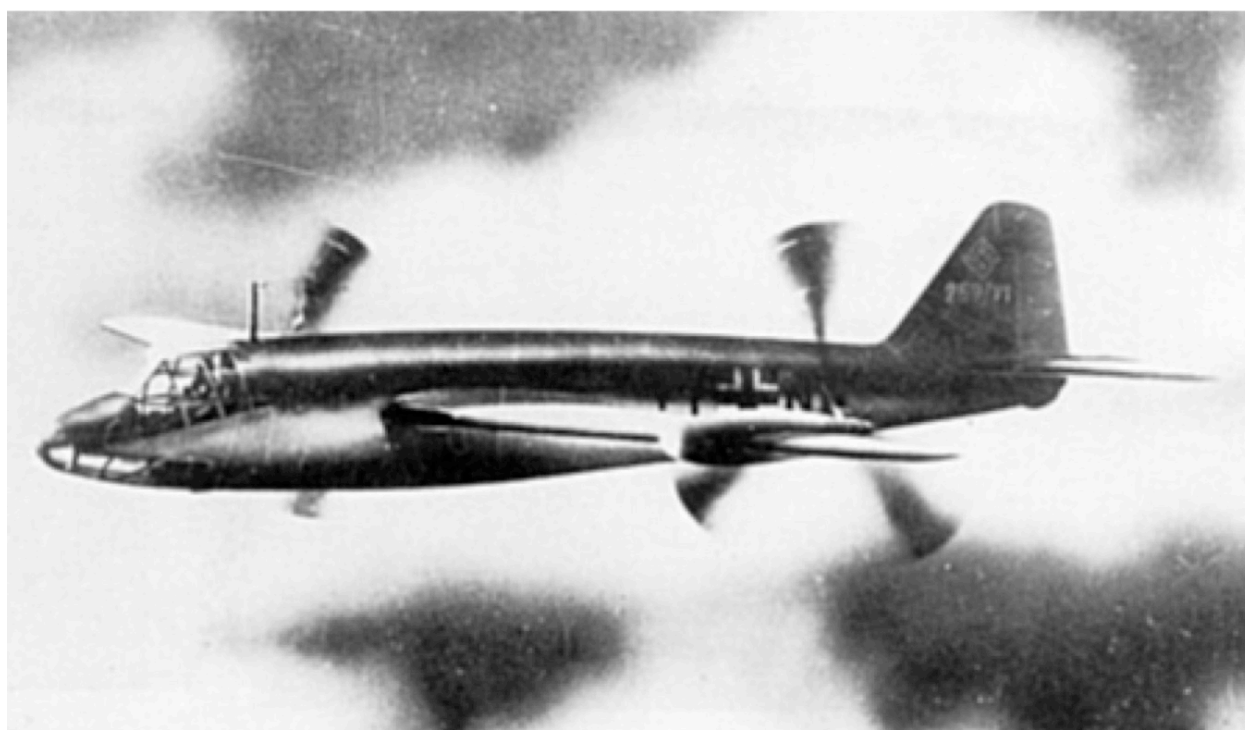
Focke-Achgelis Fa 269 tilt-rotor VTOL aircraft, designed in 1943 but destroyed by Allied bombing in 1944 (model above, drawing below)
