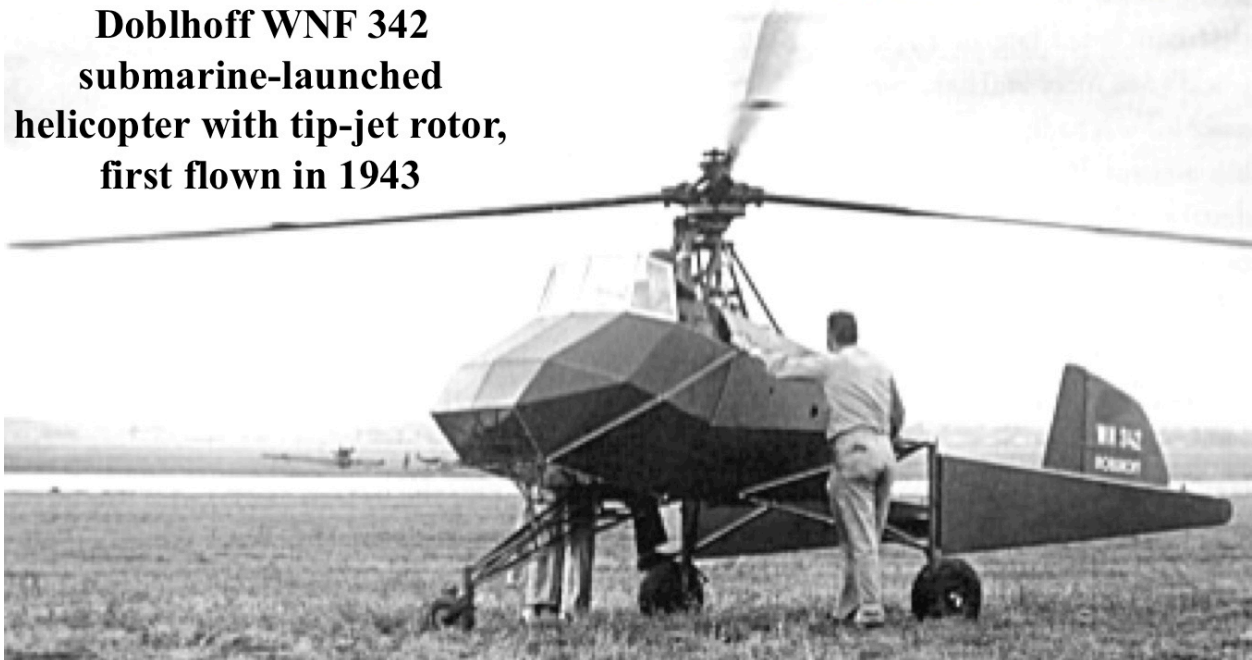
Figure 9.146: Friedrich von Doblhoff and his team including Theodor Laufer, Alexander Czernin, and August Stepan created helicopters propelled by tip-jet rotors, such as the Doblhoff WNF 342 submarine-launched jet helicopter, which was first flown in 1943.
