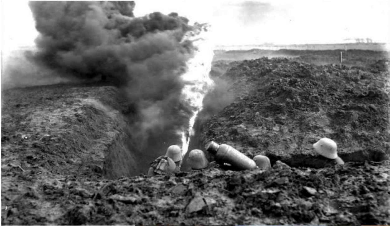
Two-person portable Kleinflammenwerfer Kleif (1912)
