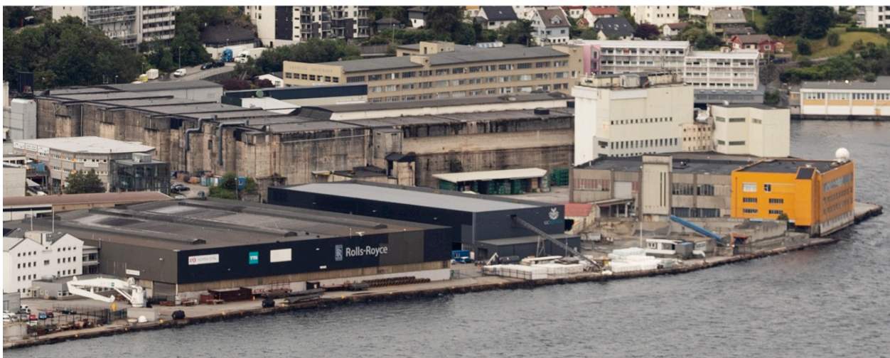
Figure 7.128: The U-boat bunker Bruno in Bergen, Norway could hold and service up to nine submarines at a time, with six meters of overhead concrete reinforcement to protect them from Allied aerial bombing.
