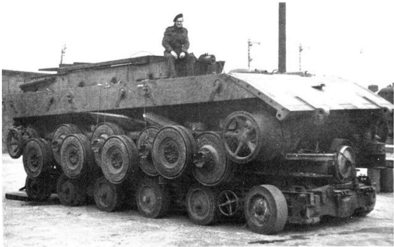
Henschel Panzerkampfwagen E-100 tank prototype (1945)
